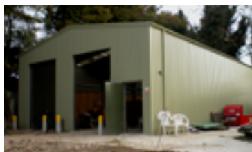
10m x 20m Machinery store
