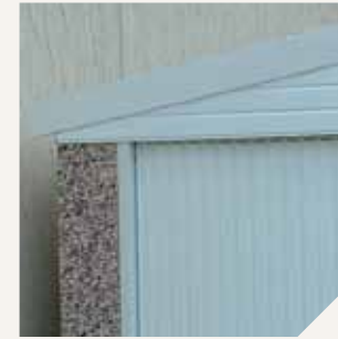
White PVCu fascias and vergeboards
